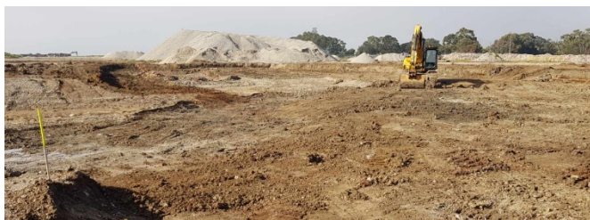
Above: Soil remediation in progress.
