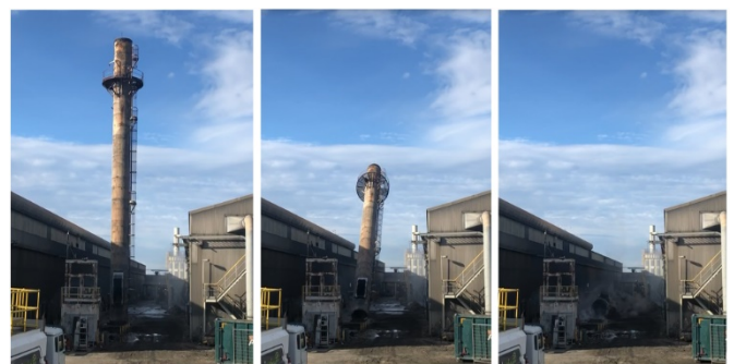
Above: The scrubber stack was felled in May.
