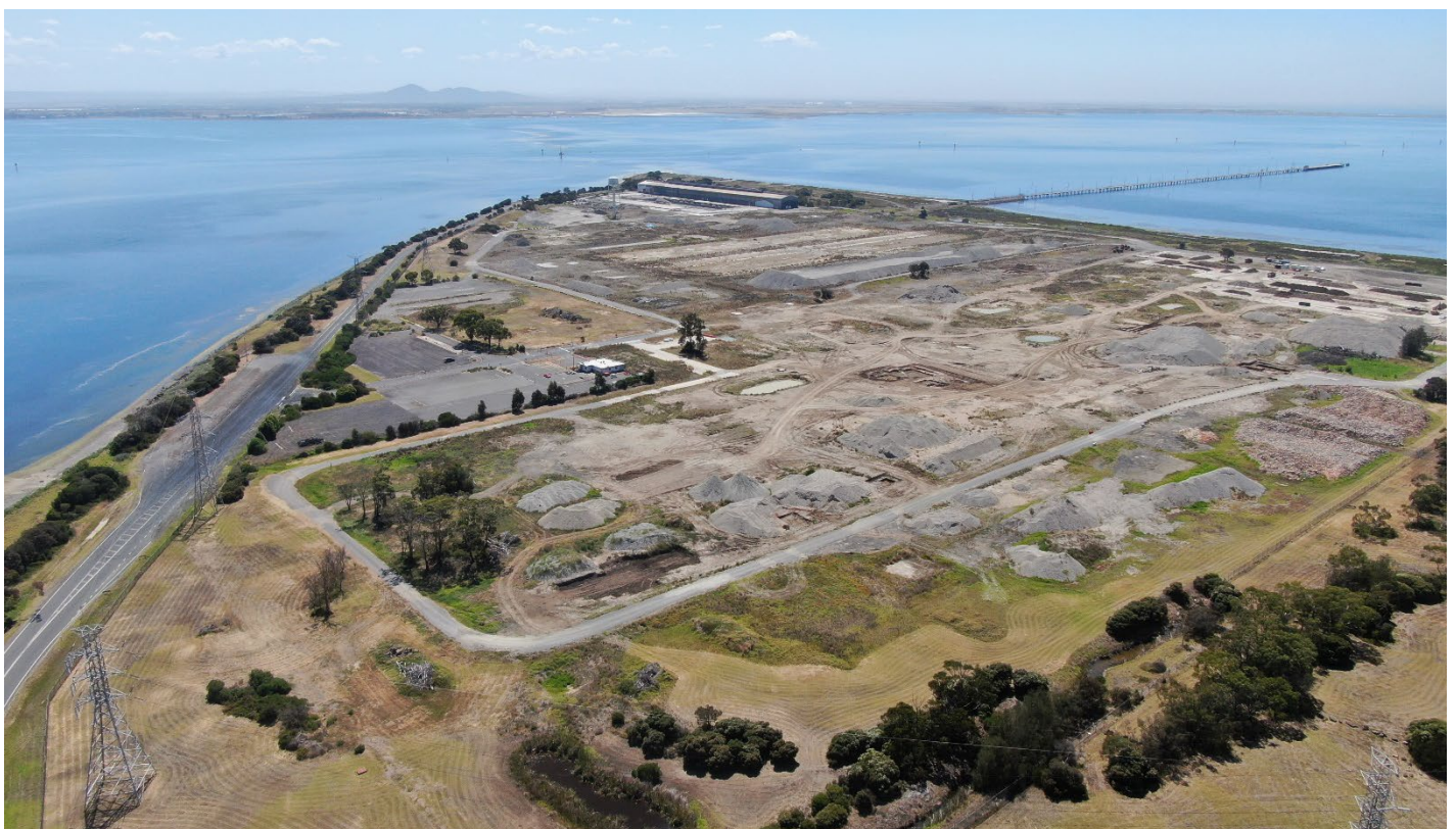
Above: The former industrial site at Alcoa Point Henry, March 2022
