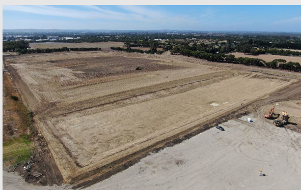
The construction of two new cells, 6 & 7, commenced in late 2021.
