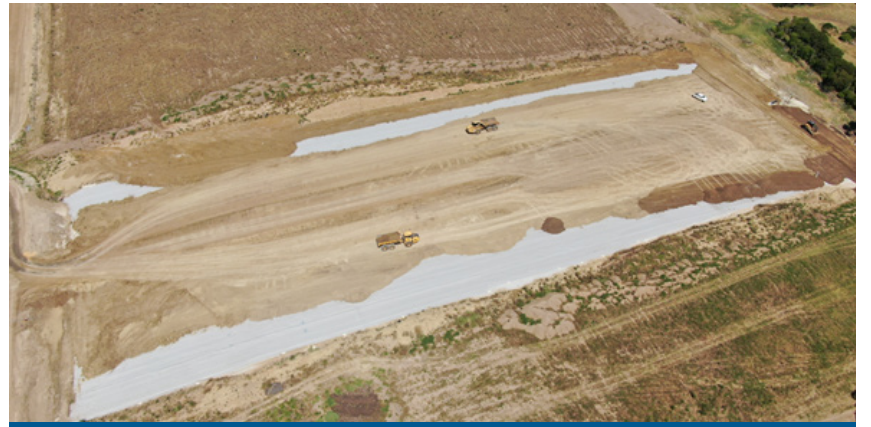
Moolap cell 6 showing best practice lining, subsoil and topsoil placement
