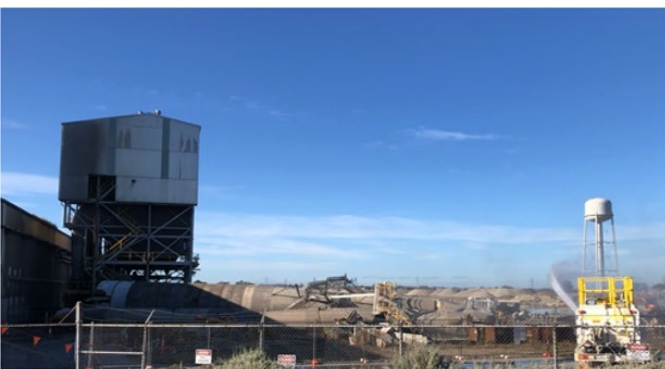
Above: The controlled collapse of the former baking furnace scrubber.
