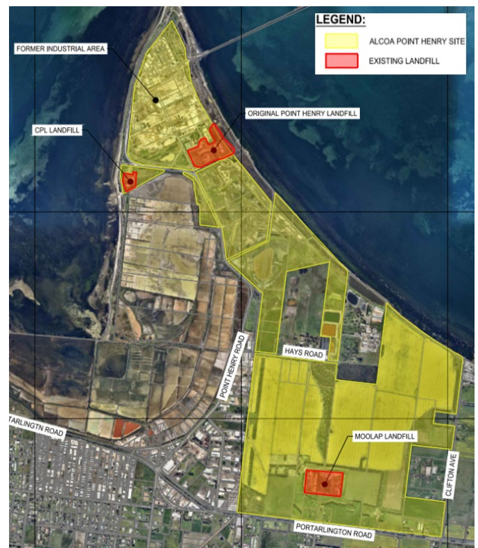
Above: Aerial photograph highlighting the three existing landfills at Point Henry.
